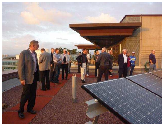
Rooftop installation on Natural Sciences II
